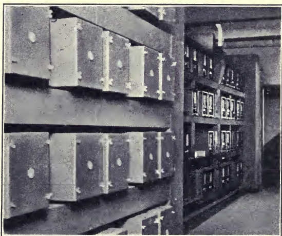
FIG. 4. Part of one of the attic reactor racks, with the reactors in place.
