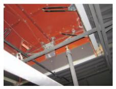
Installing a fire sprinkler below a vent is a common mistake that makes it likely that one or both will not function as intended. Also, the manual release, suitable for use on a 20' warehouse roof, is frequently inaccessible to occupants on a stage.
