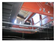
This vent is motorized with easy operation from the floor for emergency and testing use. Unfortunately, the vent with this factory option is not labeled.
