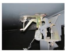
Computer modeling shows that a fusible link mounted on the vent will not open until well after the audience has left the auditorium. This vent has been modified for stage floor operation, which has nullified the conditions of it being labeled.
